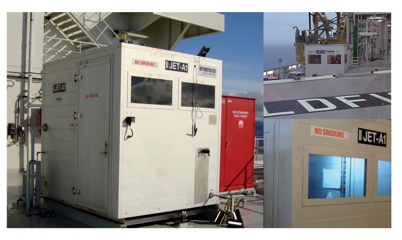
Can be delivered with standard equipment or be upgraded to project specific requirements This walk-in and operator preferred unit can be delivered with standard equipment or be upgraded to project specific requirements. Our Walk-in Dispenser Unit is an upgraded version of our standard Dispenser Unit and fulfills all requirements for Helicopter Fuelling Systems worldwide. Our design complies with all international regulations. Most common are DNV, ABS, Lloyd, RMRS, CAP 437, NOG and OSCG.
