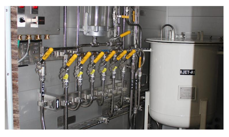
The cabinet is connected to the fuel storage tank and dispenser unit by solid pipes
