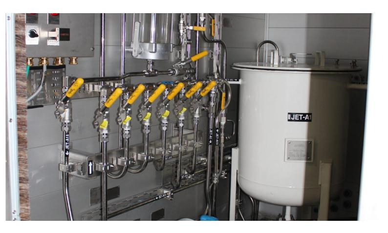
The fuel can be sampled in a closed system, avoiding spill and unsafe operation
